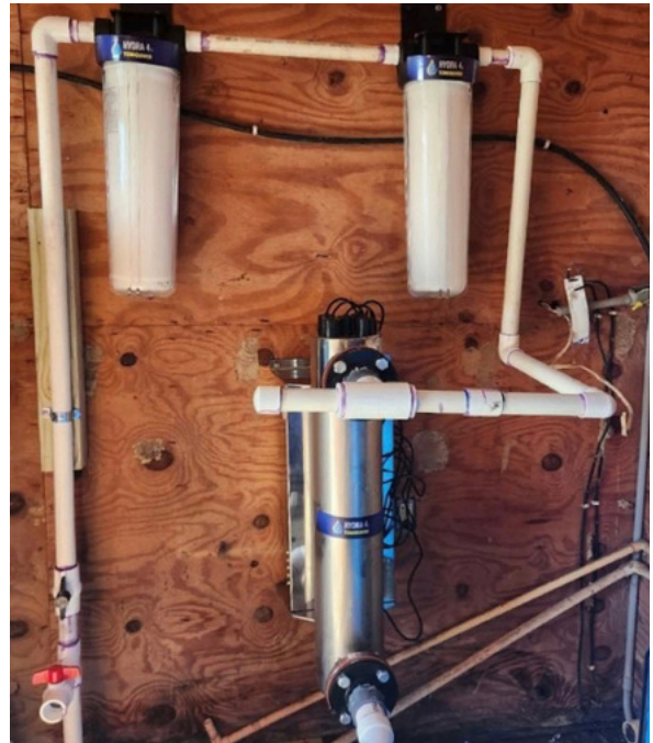
HYDRA by TOMIGUNN combines fine-fabric prefiltration and ultraviolet purification.
