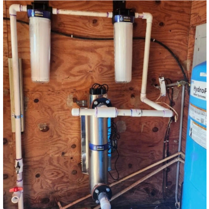
HYDRA filtration combines natural mineral prefiltration and ultraviolet purification.
